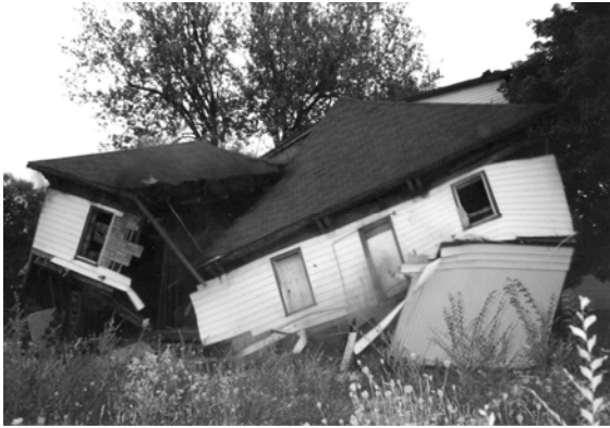
The middle interior beam is pulled out and the Union Jack collapses
